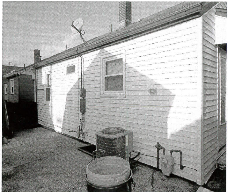
Rear View Date Taken:12/05/2012
